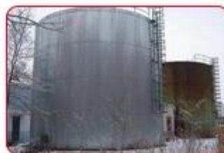
Water level measurement
